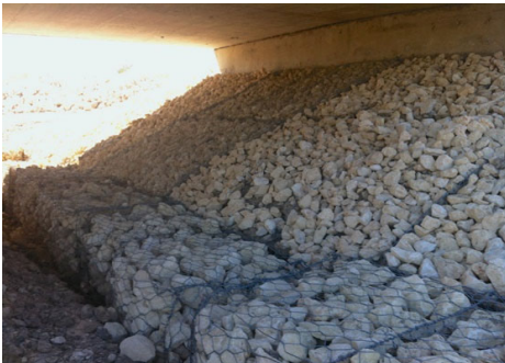
The City places riprap under bridges to protect the structure from erosion
