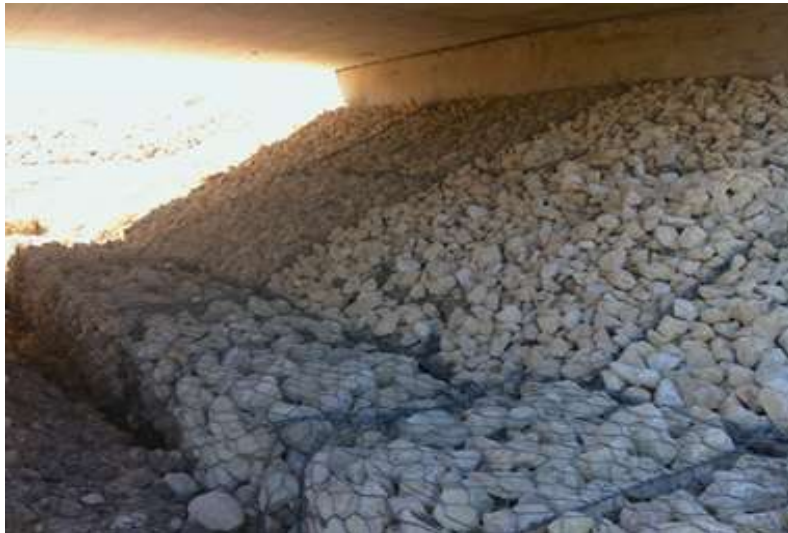
The City places riprap under bridges to protect the structure from erosion
