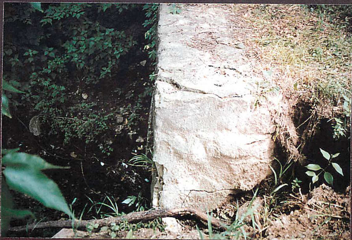
Looking at lowered channel U/s of stone arch culvert
