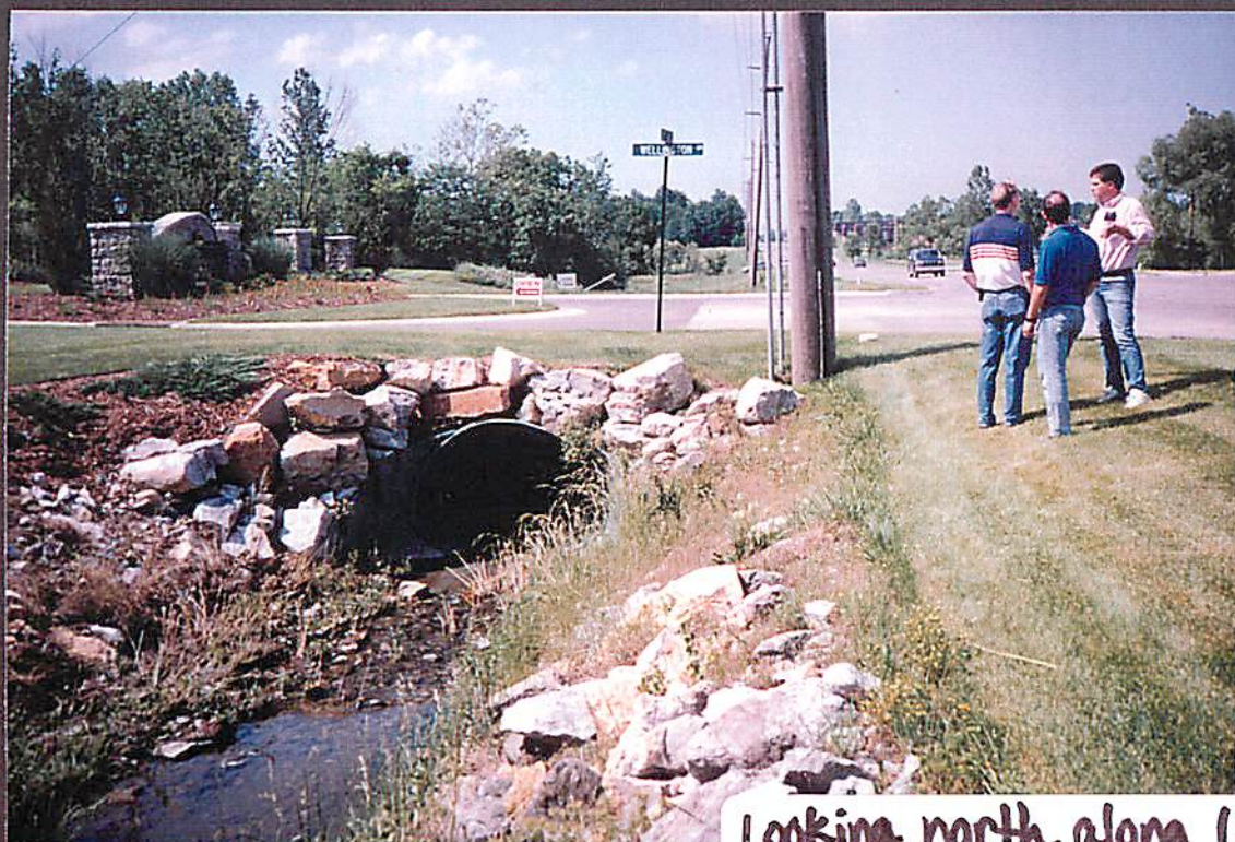
Looking south along 10th U/s of Wellington culvert. Creek can't make left turn during flood + jumps to 10th
